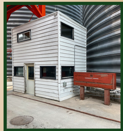
Scale House Exterior
